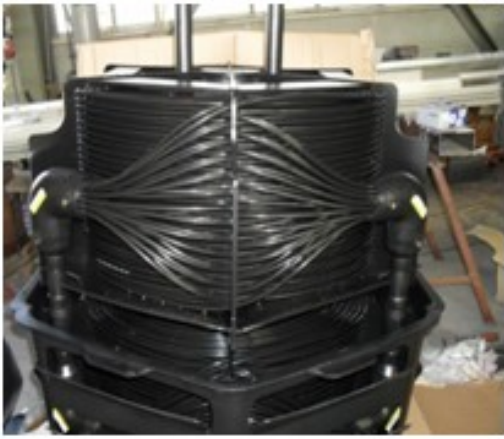
Fig. 12: “Compact” heat exchanger without envelope
