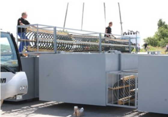
Fig. 14: Process of constructing of two spirals- heat exchanger between of three parts of pontoons
